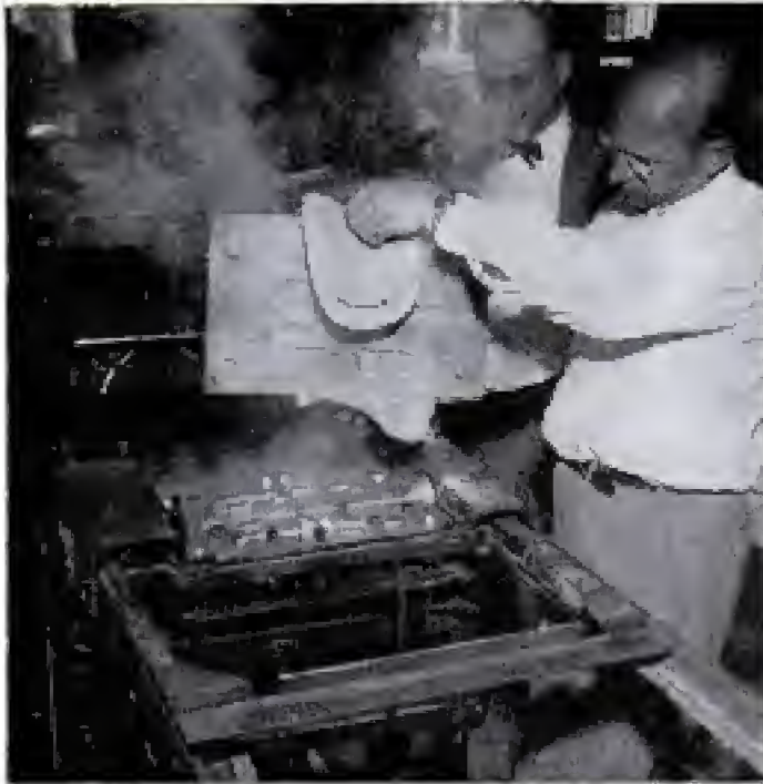
Left, new shell mold is taken from machine. Right, casting from matched plastic molds is clean and smooth
